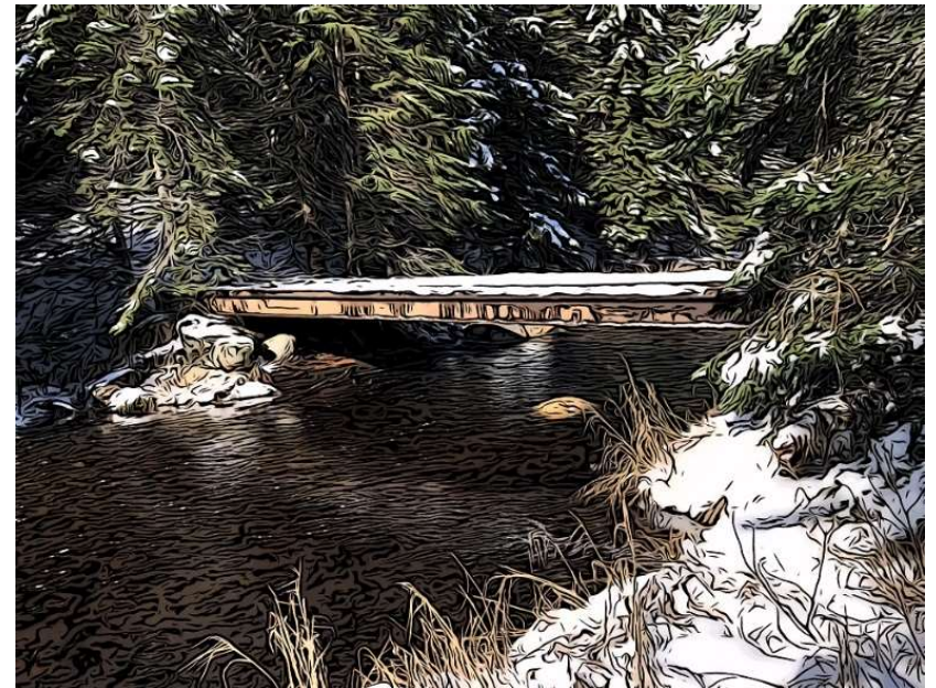
Small bridges can save a lot of grief if shallow soils limit culvert size
